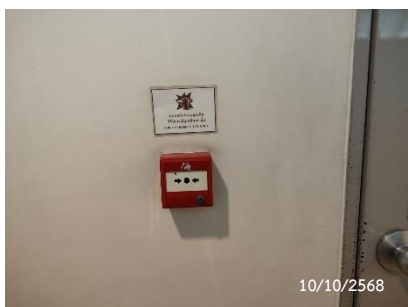
Fire Alarm Manual Call Point
