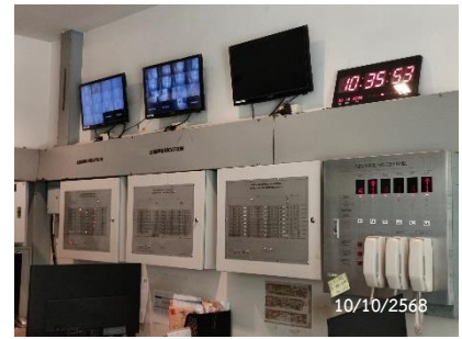
Graphic Annunciator Fire Alarm System
